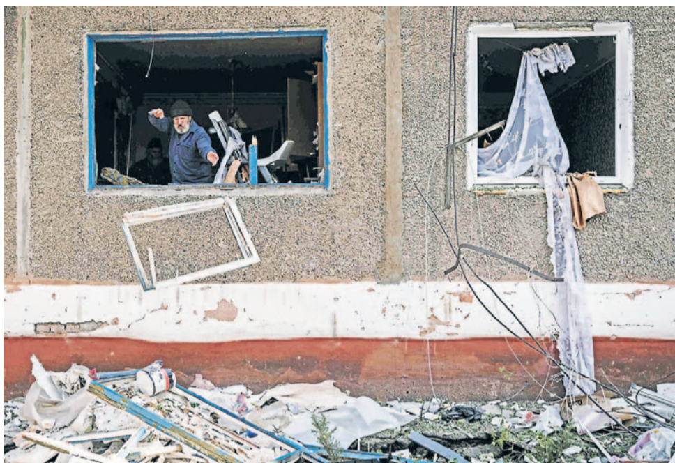
An apartment damaged by a missile in Kramatorsk, eastern Ukraine, on Thursday.
