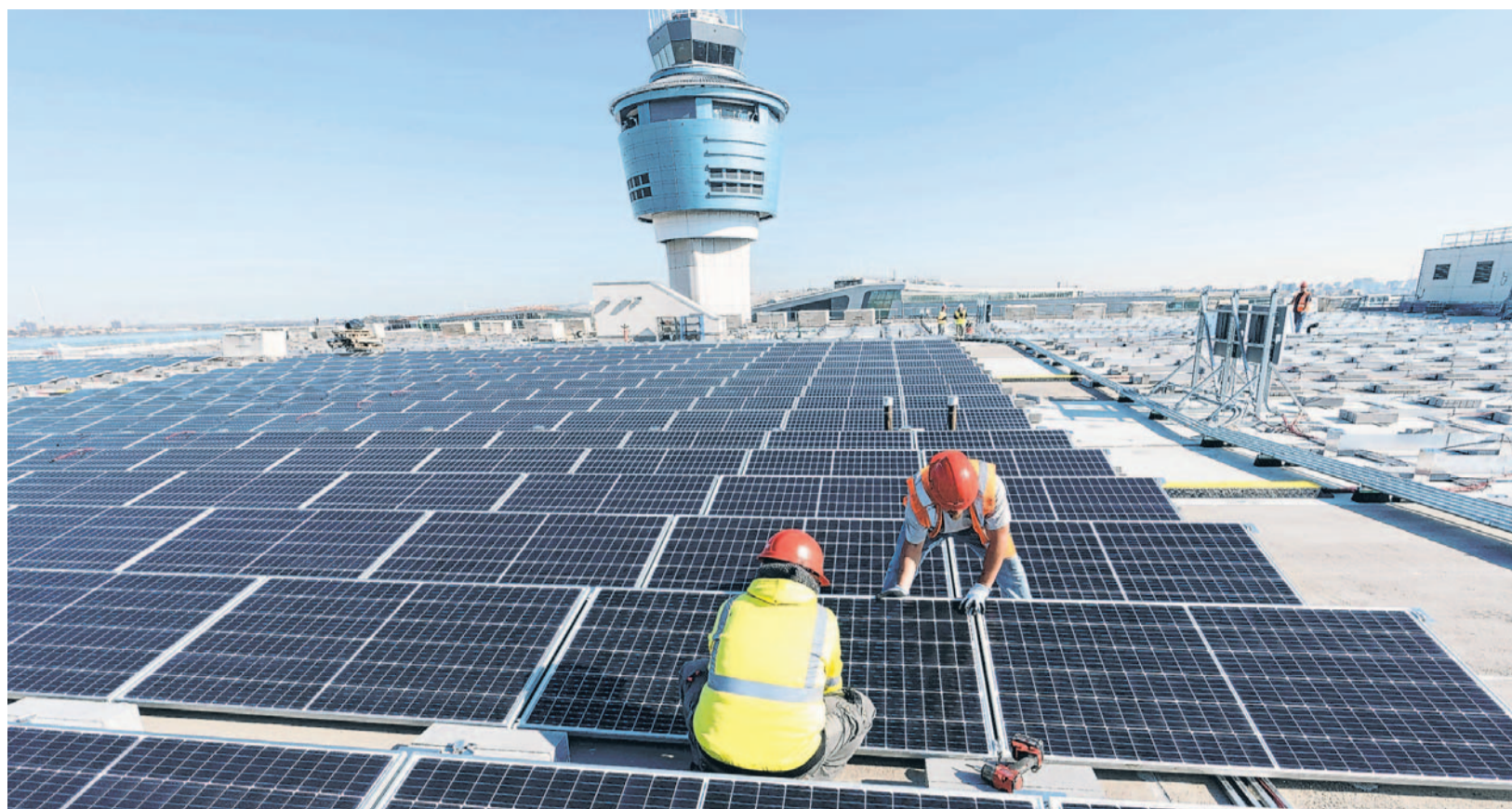
Solar panels at LaGuardia Airport in New York City. Cambodia, Thailand, Vietnam and Malaysia produce roughly 80% of solar modules imported into the U.S.
