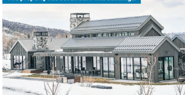
The property has seven barn-like buildings.
