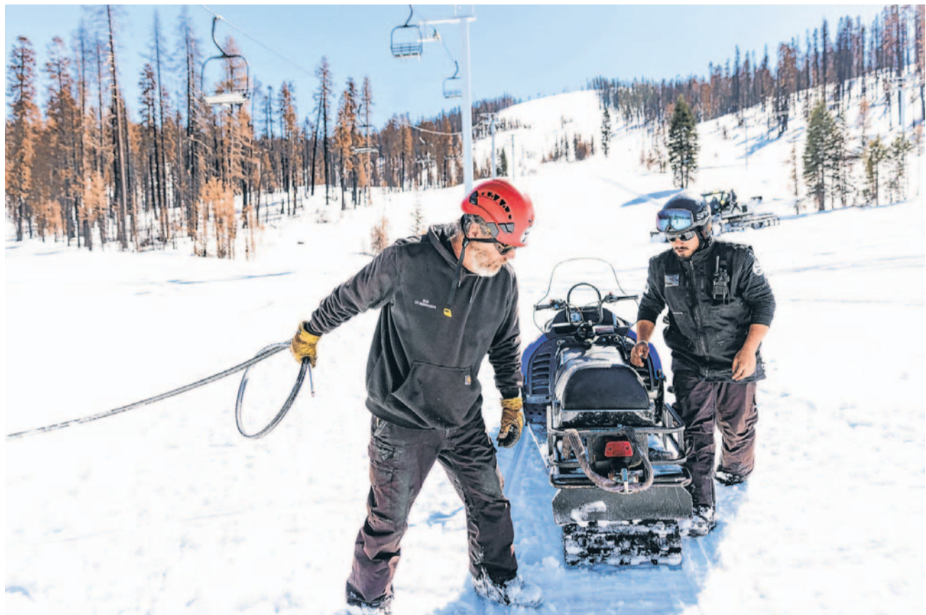
Sierra-at-Tahoe Resort electrician Bob Dean, left, and mechanic Joe 'Snowball' Hanania remove equipment damaged by a wildfire last year.
