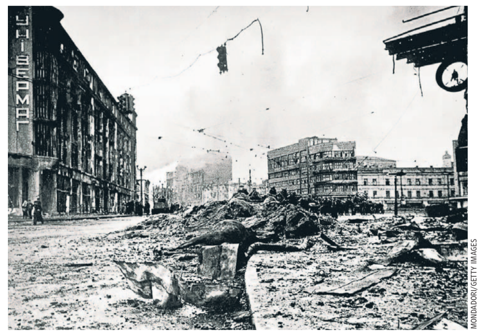
The damage to Kharkiv in the aftermath of the German assault.
