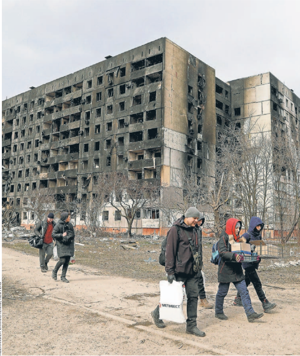
In Mariupol, Ukraine, people on Thursday walked past a residential building that was bombed by Russia. A local official said 80% to 90% of the city has been destroyed.
