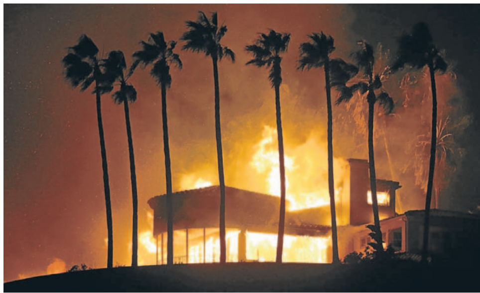
A Malibu home ablaze in 2018. Fires are driving some insurers out of California’s high-end market.
