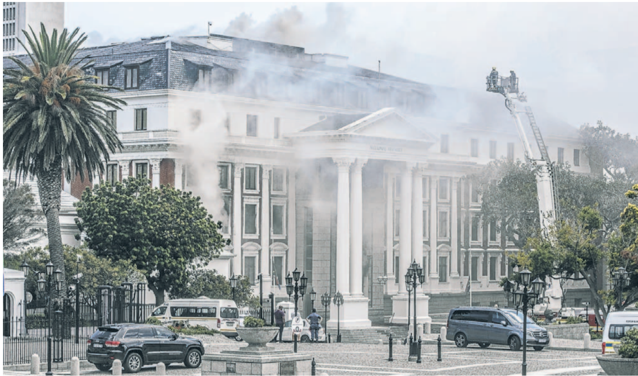
More than 70 firefighters in Cape Town on Sunday battled a blaze at South Africa's parliament building, the government's main working legislative venue and part of a designated heritage site in the city center. The ceiling at the National Assembly collapsed.
