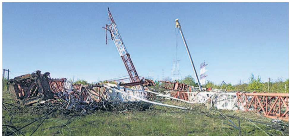
Soviet-era radio towers that broadcast Russian-language stations were damaged after explosions in Transnistria. Photo was issued by the breakaway region's interior ministry on Tuesday.
