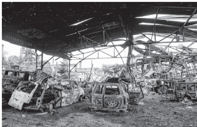
Destruction at a steel plant in Mariupol, Ukraine, last week.
