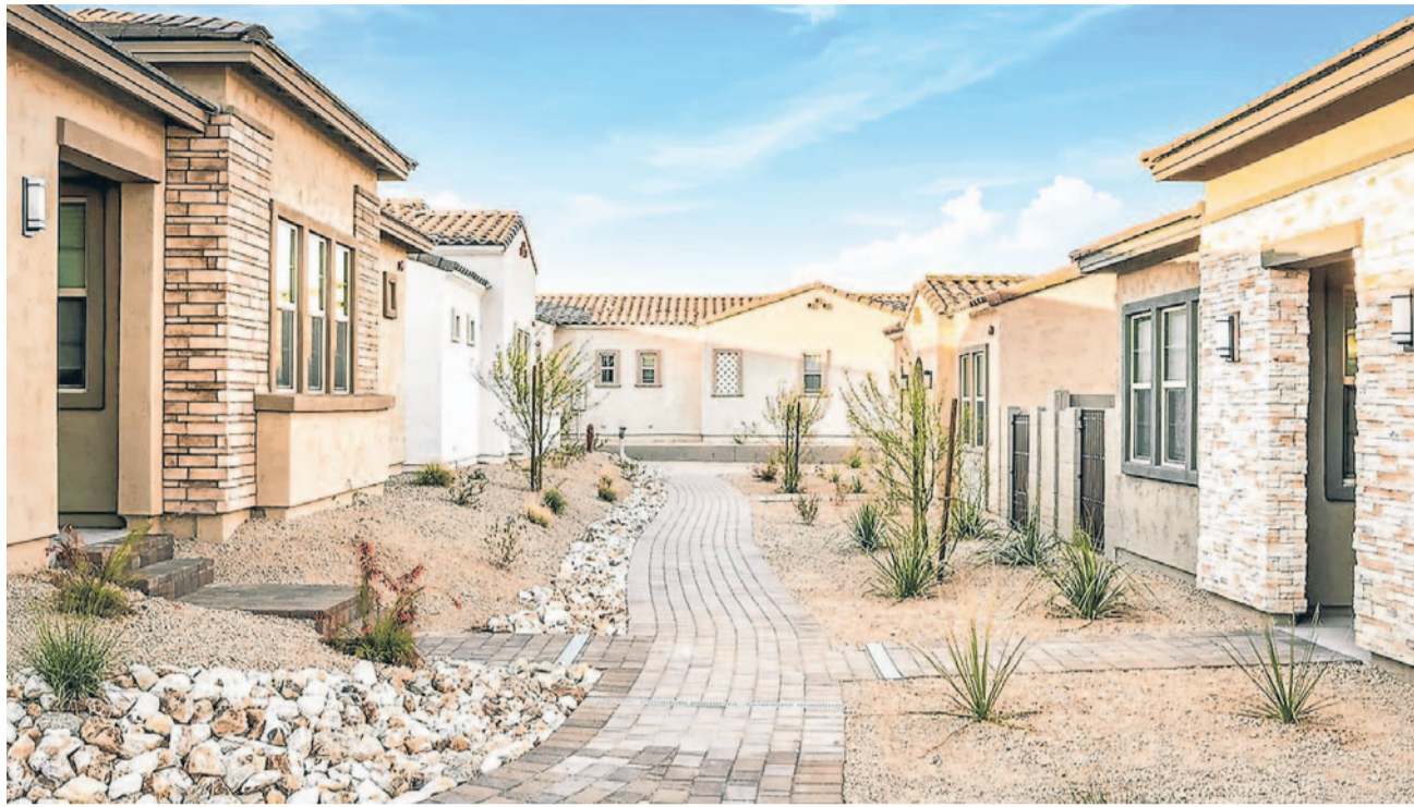
Houses in Havenly Fountain Hills, a community about 30 miles outside of downtown Phoenix, where homes rent for more than $2,500 a month, which allows the company to ride out headwinds in the for-sale market. Below, a common area of the clubhouse and leasing office.
