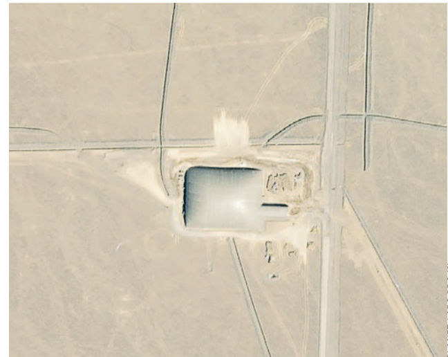
Construction in June 2021, top, near Yumen, China, of a site believed to be set to become one of 120 silos to hold nuclear missiles. Work appears to progress the following month, bottom.
