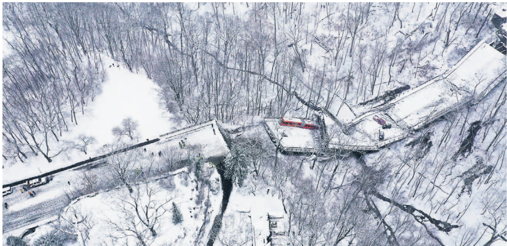
A 50-year-old Pittsburgh bridge collapsed Friday, injuring 10 people. The 450-foot-long span was graded as poor in inspections from 2011 through at least 2017.
