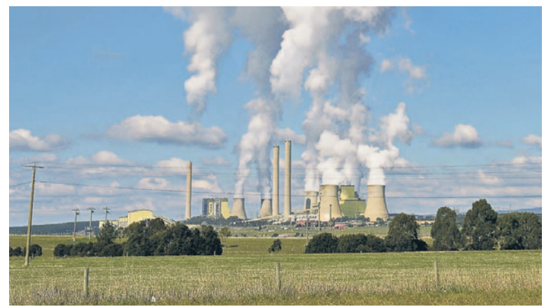
A power station operated by AGL Energy in the Latrobe Valley, Australia.
