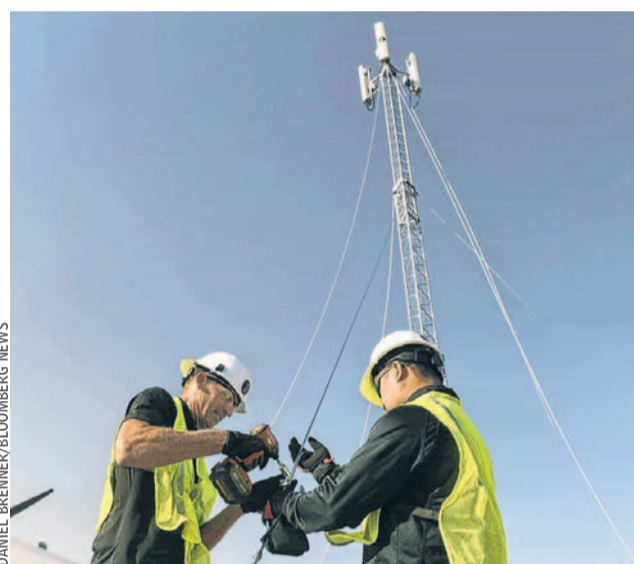
Technicians set up a Dish portable wireless tower in Colorado.
