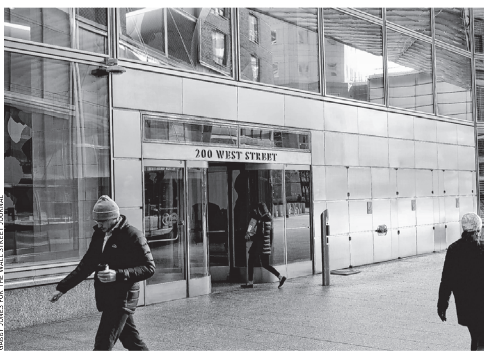
Goldman Sachs requires vaccines for workers and visitors. Its building is in Lower Manhattan.
