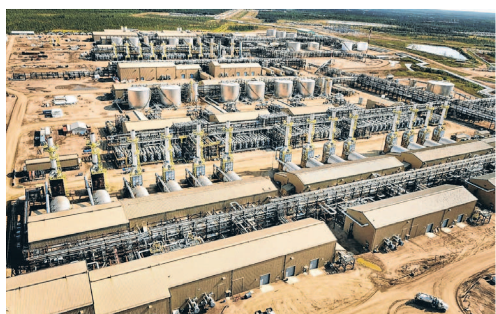
A processing plant at Cenovus Energy’s Christina Lake oil sands project in northern Alberta.
