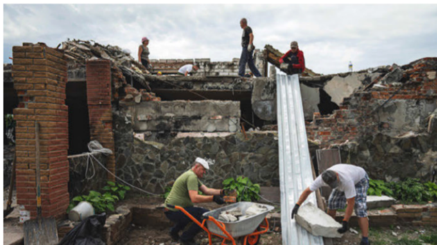
Another few bricks in the wall
