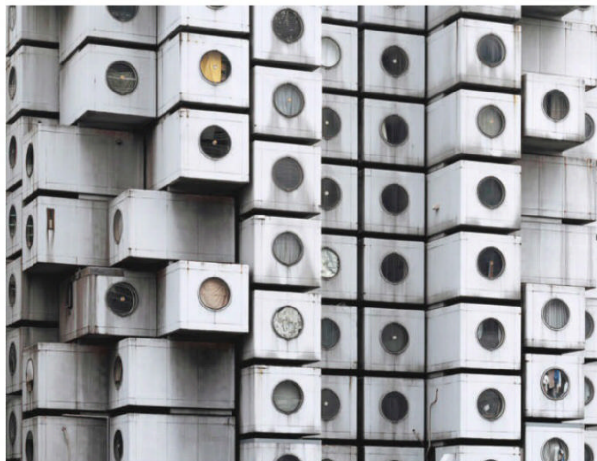
Chipping off the old block
